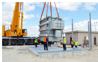
Transformer installation (courtesy US Army).
